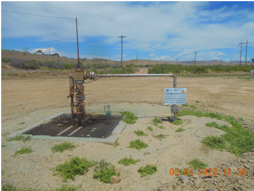
Injection wellhead.
