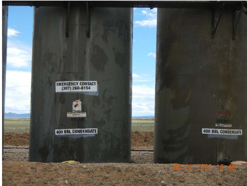
Photo 5. Incomplete tank labels.
