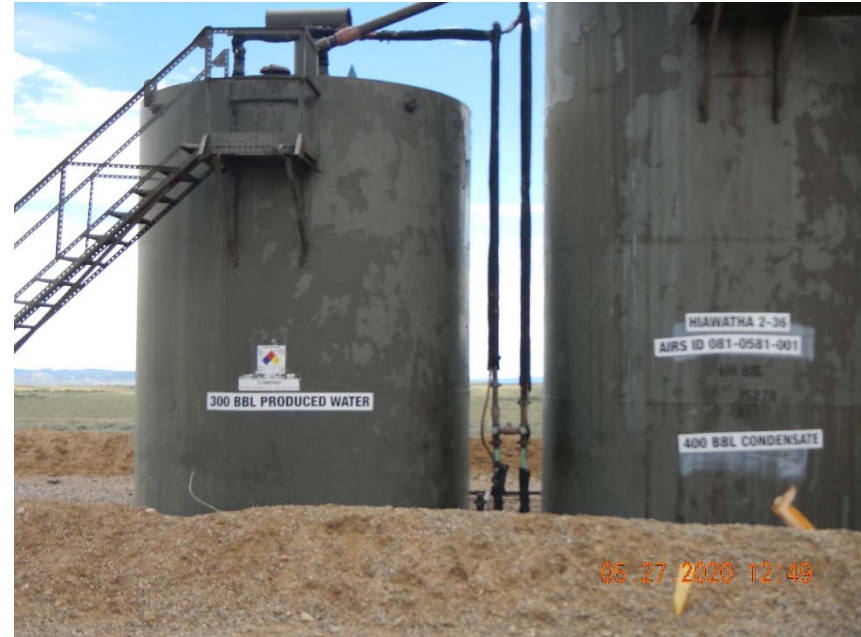
Photo 6. Incomplete tank labels.
