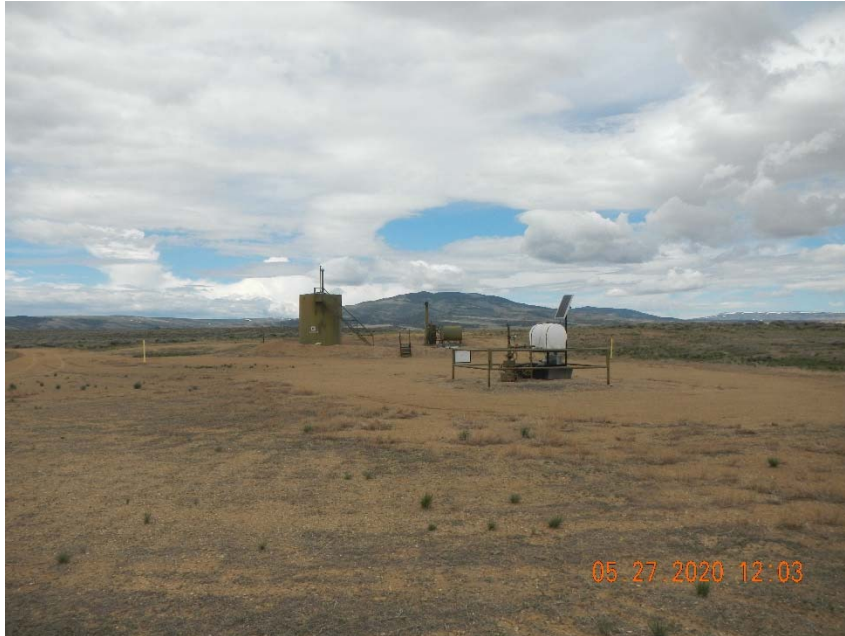
Photo 1. Overview of location taken facing west.
