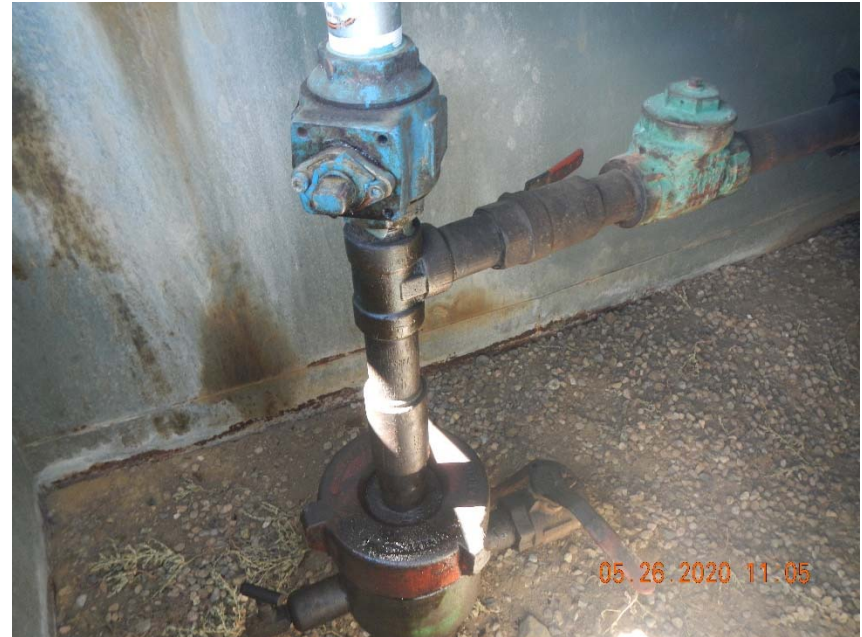
Photo 2. Photo of wellhead inside housing.
