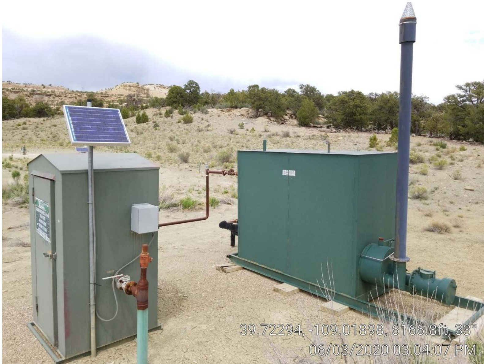
Photo 3. Meter building & separator.
