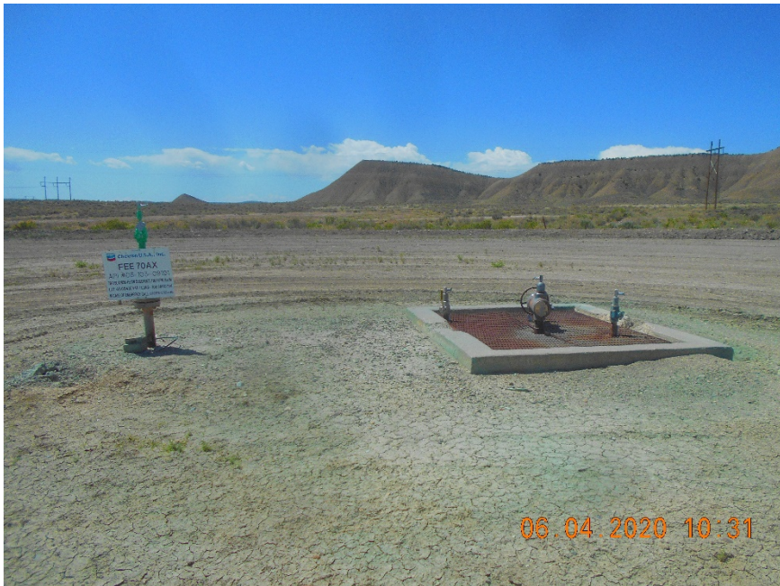
Injection wellhead. Temporarily Abandoned
