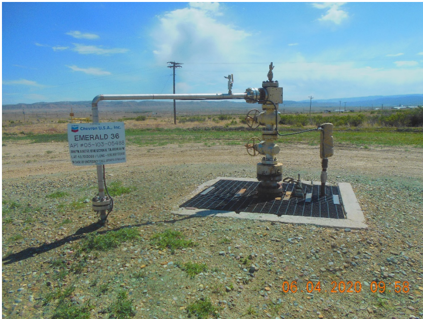
Injection wellhead.
