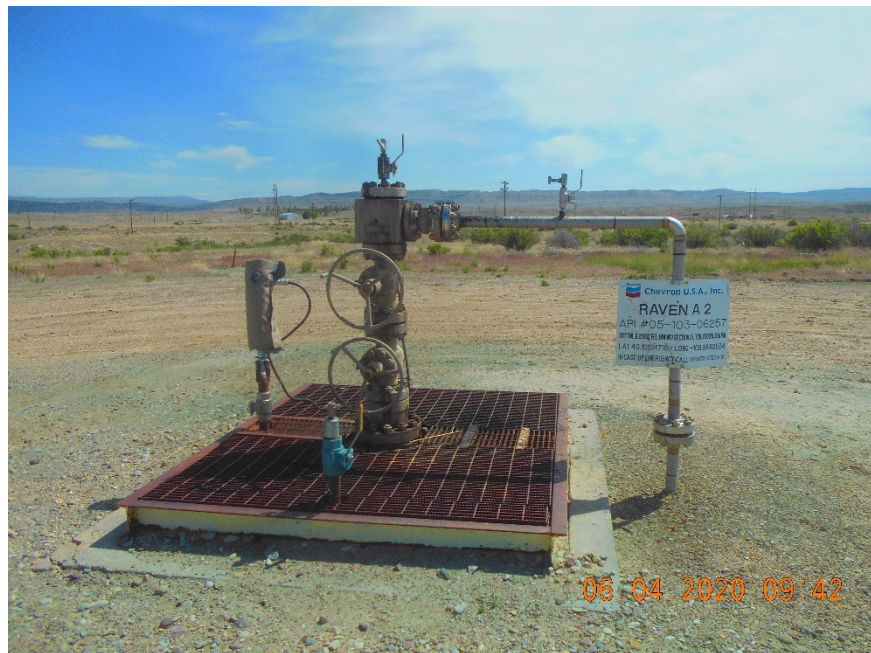
Injection wellhead.
