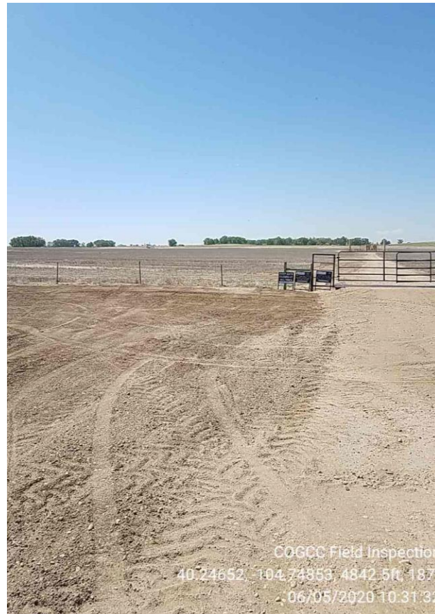
Photo 1 Photo of Area Where Riser Has Been Removed.
