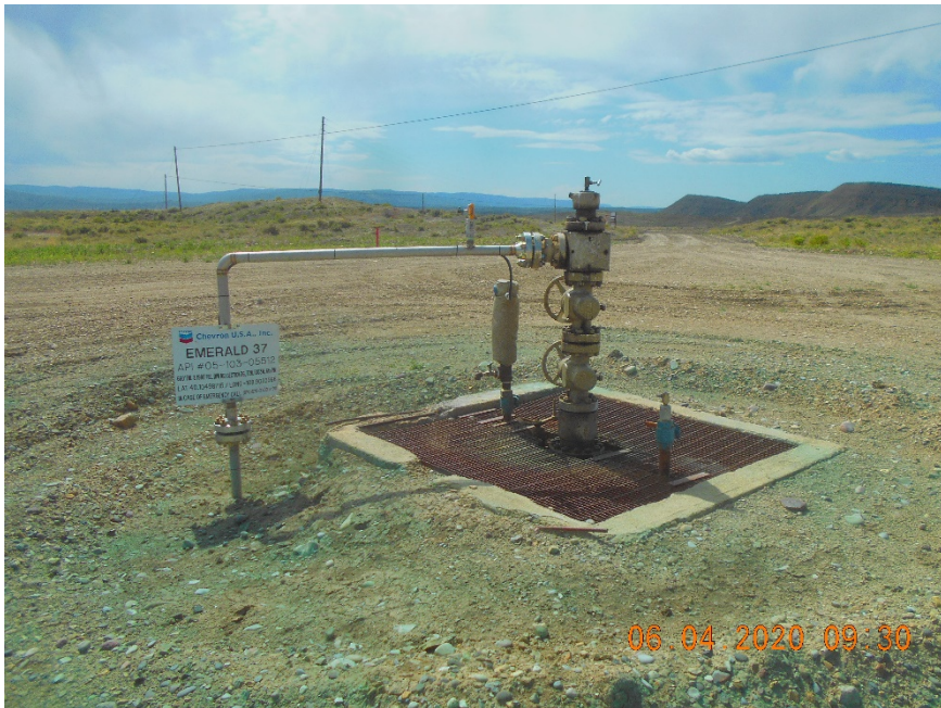
Injection wellhead.
