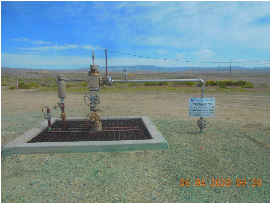
Injection wellhead.
