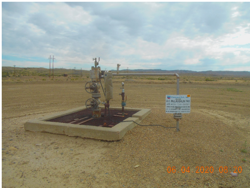
Injection wellhead.
