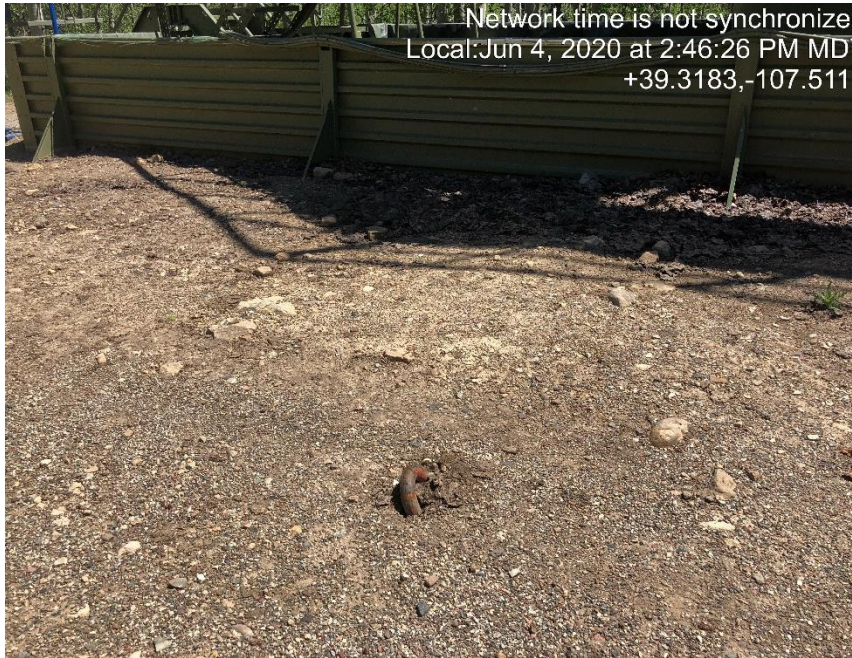
Photo #1319 Deadman not properly marked.
