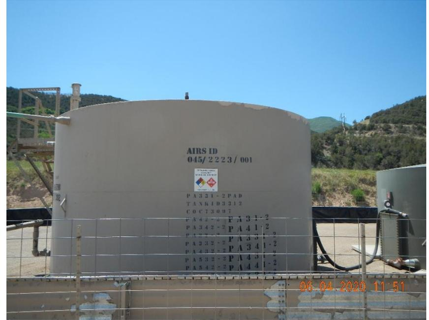
**Tank capacity too small to read at distance.**
