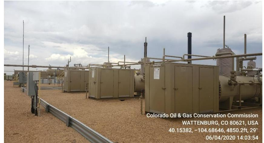
**Photo 5 Horizontal Heated Separators**
