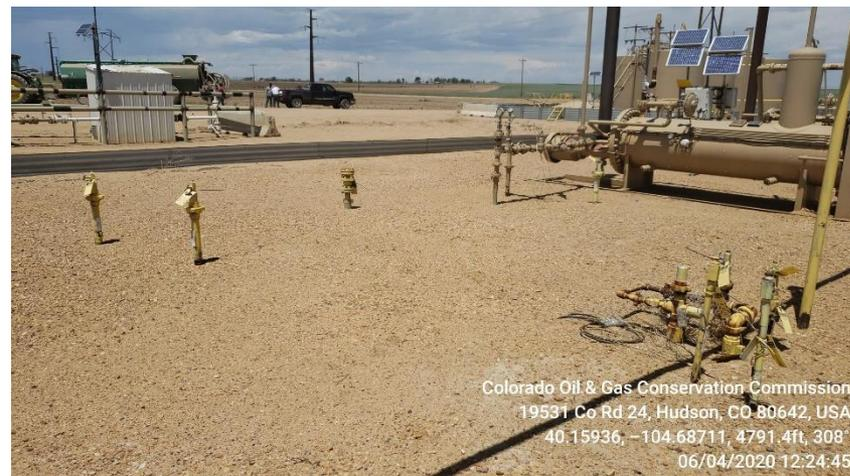
**Photo 3 Horizontal Heated Separators and ECDs**
