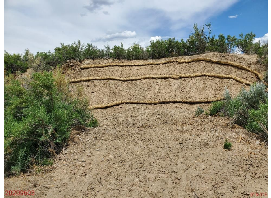
Photo 4: Photo taken from the Location, facing east. Photo shows BMPs installed on slopes.
