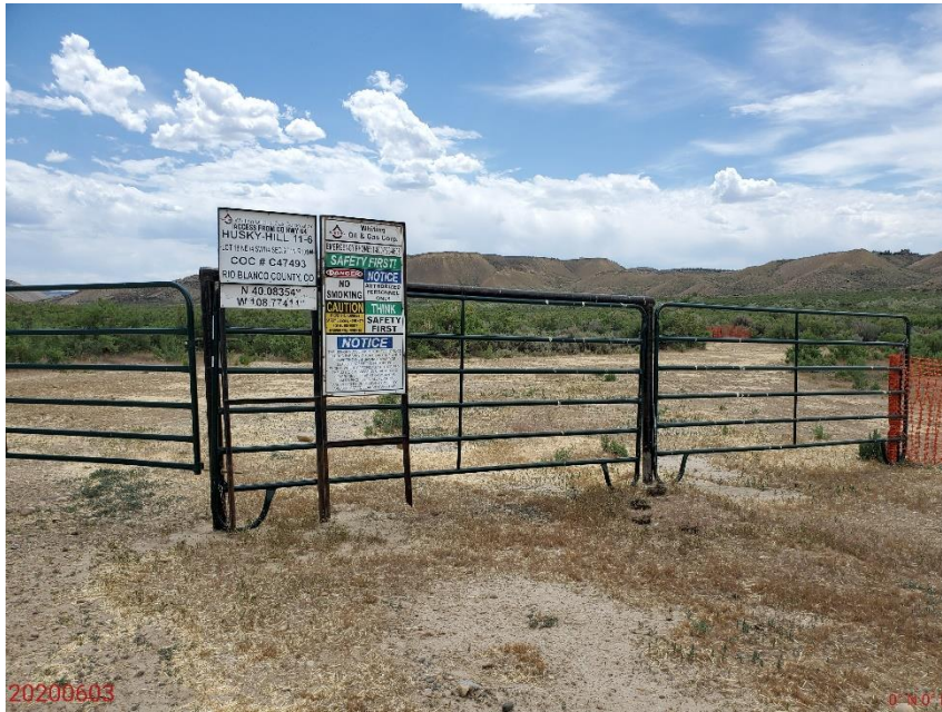
Photo 1: Photo taken from the access road. Photo shows additional fencing and signage has been installed.
