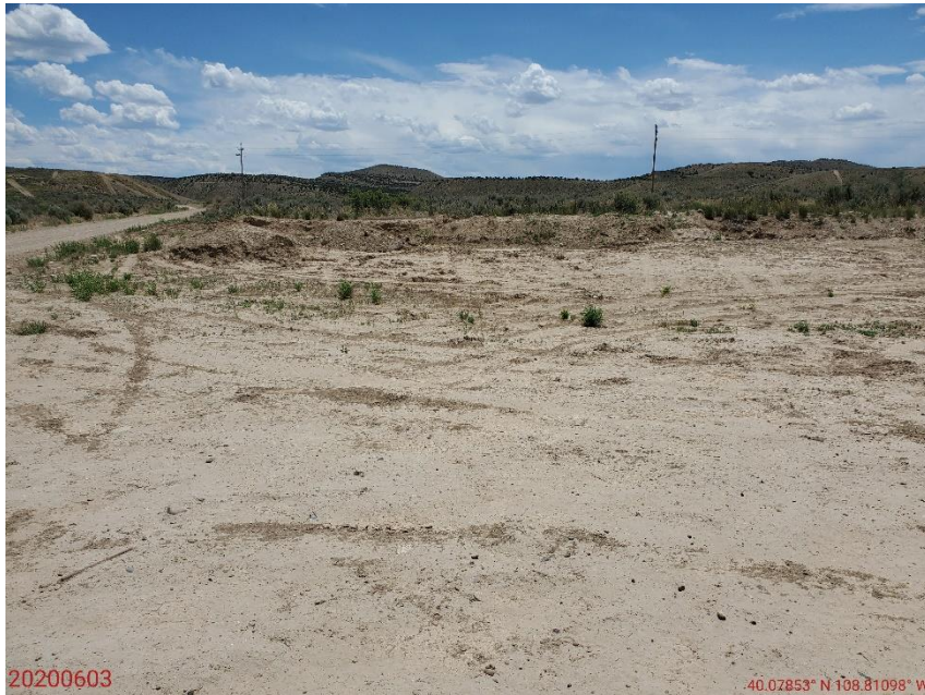
Photo 1: Photo taken from the east end of the Location, facing south. Photos 1-4 provide an overview of the Location from south, southwest, northwest to north. Photo shows equipment and debris has been removed from the Location. Photo also shows no additional reclamation activities appear to have been conducted pursuant to Rule 1004.a and corrective actions.
