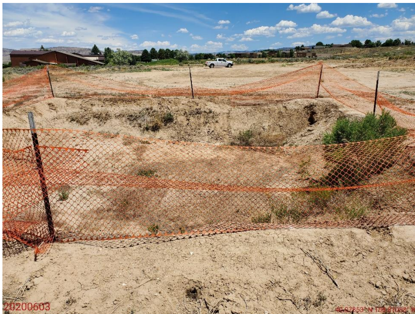
Photo 7: Photo taken from the west side of the pit, facing east. Photo shows pit has not been closed; Pit closure in process.
