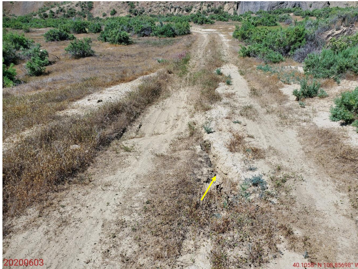
Photo 5: Photo taken from the northern access road, facing west. Photo shows stormwater erosion remains evident; No BMPs appear to have been installed.
