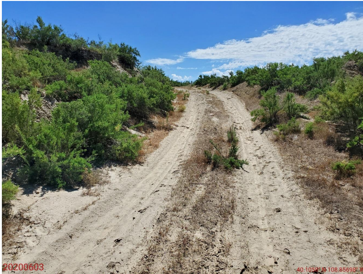
Photo 12: Photo taken from the southern access road, facing south. Photo shows access road has not been contoured or regraded.
