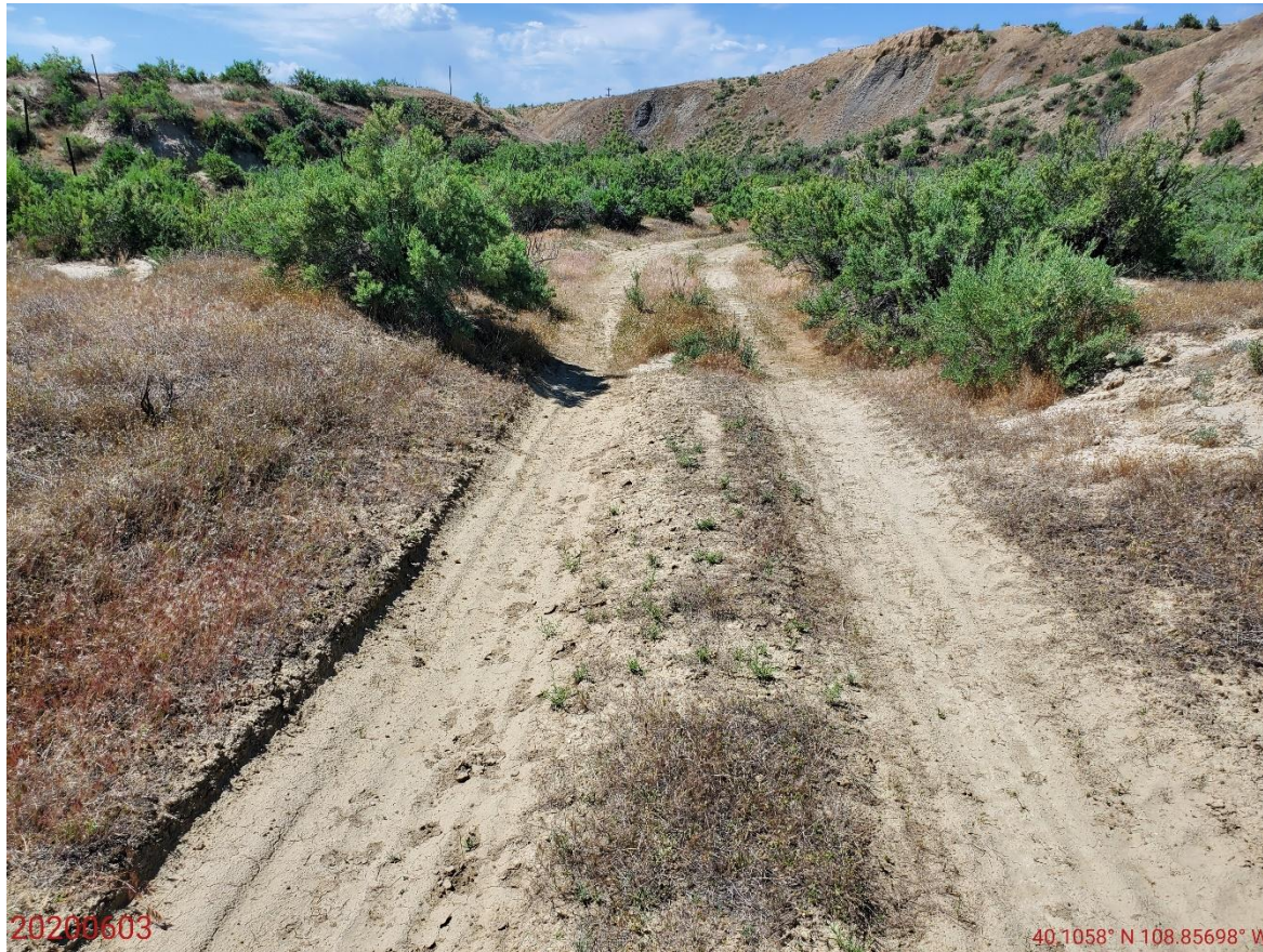
Photo 6: Photo taken from the northern access road, facing west. Photo shows access road has not been contoured or regraded.
