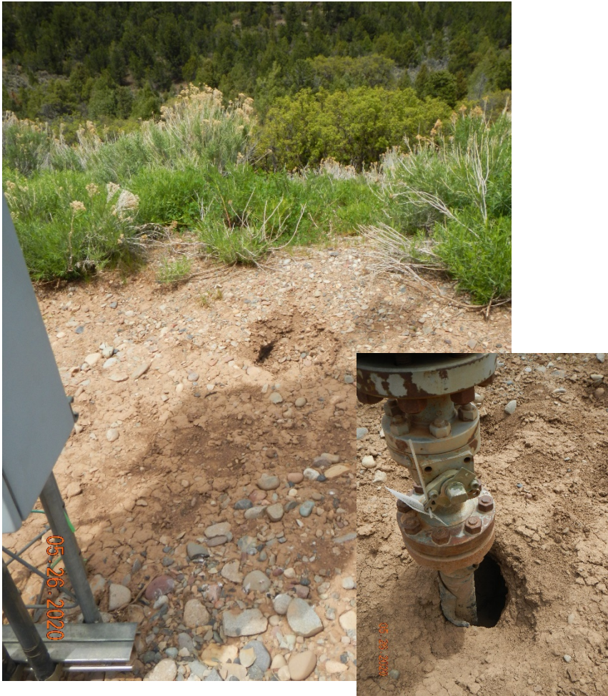
Photo#2: Erosion tunneling.
