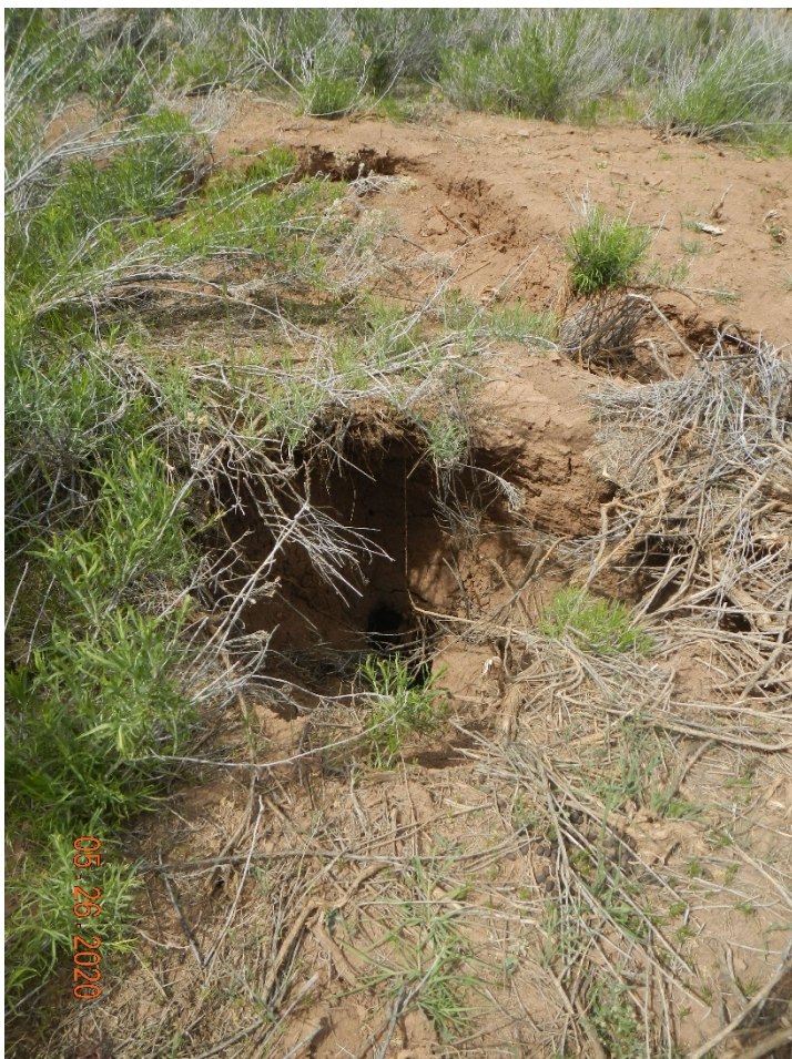
Photo#4: Daylighting and subsidence further down the fill slope.
