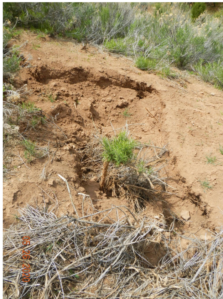
Photo#5: Daylighting and subsidence further down the fill slope.
