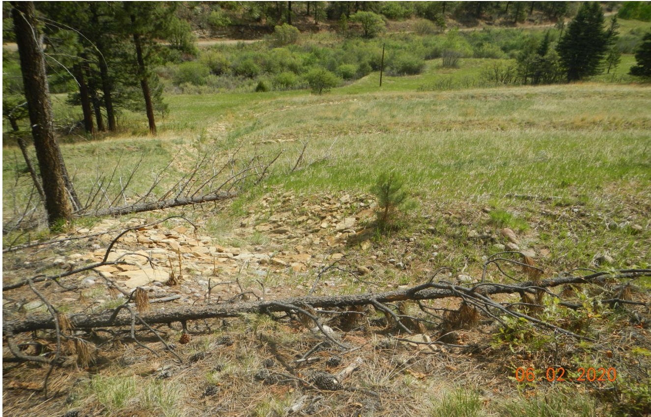
Photo 9. Facing northeast at the location. The upper run-on ditch and berms are directed toward the riprap drainage area. No stormwater issues were observed.
