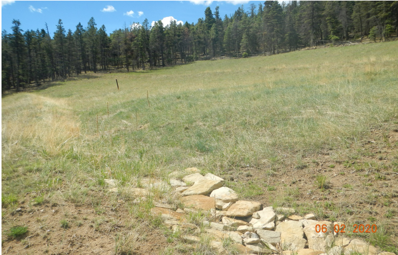
Photo 5. Facing southeast toward the location. There is a berm installed along the contour of the slope with rock rip/rap outlet protection. Berm can be seen In left side of photo.
