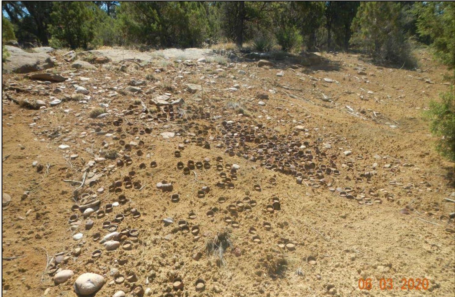
Photo 5. View of numerous metal rings that appear to have been exposed from erosion on the well pad cut-slope. Debris needs to be removed. Cut-slope needs stabilization.
