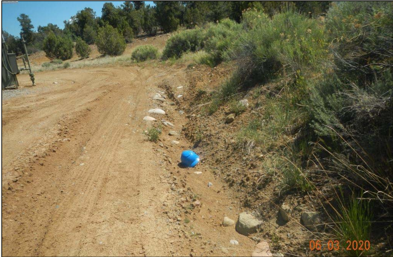
Photo 4. View of erosional channel at the well pad entrance, approximately 18 inches wide and deep (hard had in place for scale). Area of erosion was identified during 2016 reclamation inspection.
