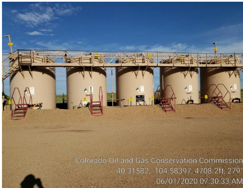
Photo #3 Tank Battery
