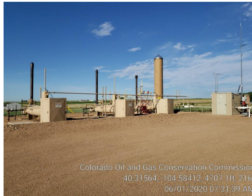
Photo #4 Separators, ECD & Meter Runs
