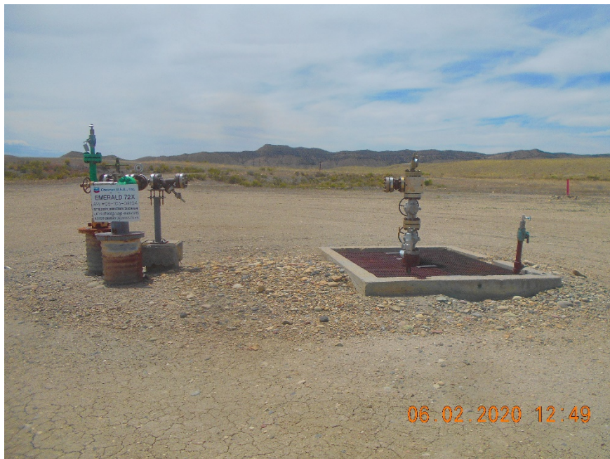
Injection wellhead. Temporarily Abandoned.
