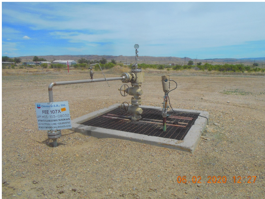
Injection wellhead.
