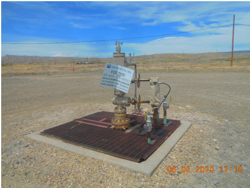
Injection wellhead.
