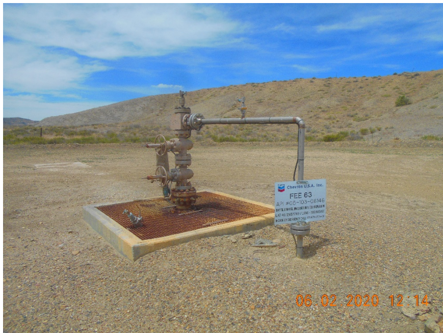
Injection wellhead.
