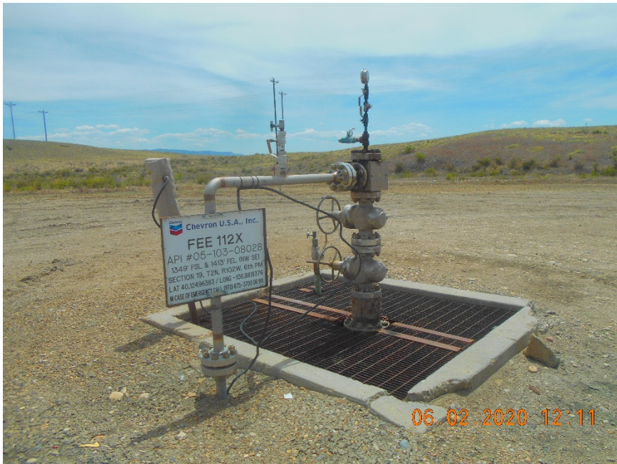
Injection wellhead.
