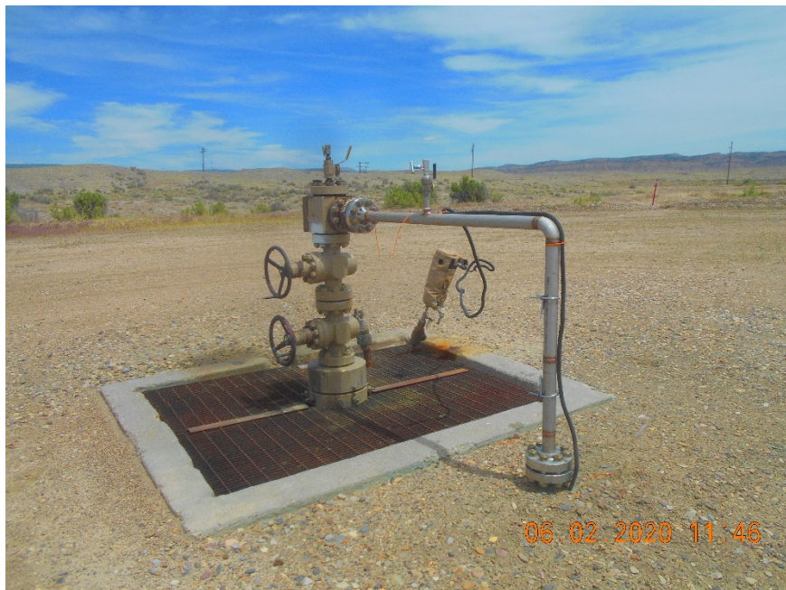
Injection wellhead.
