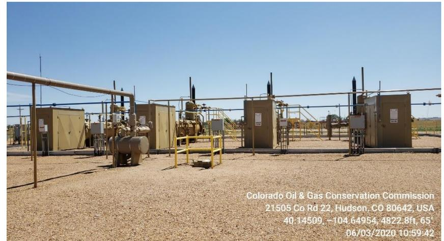
**Photo 13 Horizontal Heated Separators**
