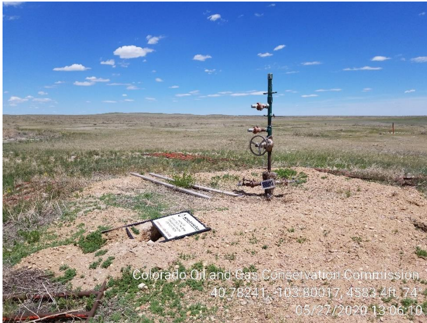
Photo 1 – Wellhead – Weeds actively growing and Fencing is in disrepair
