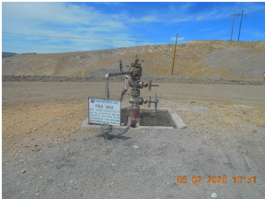
Injection wellhead.
