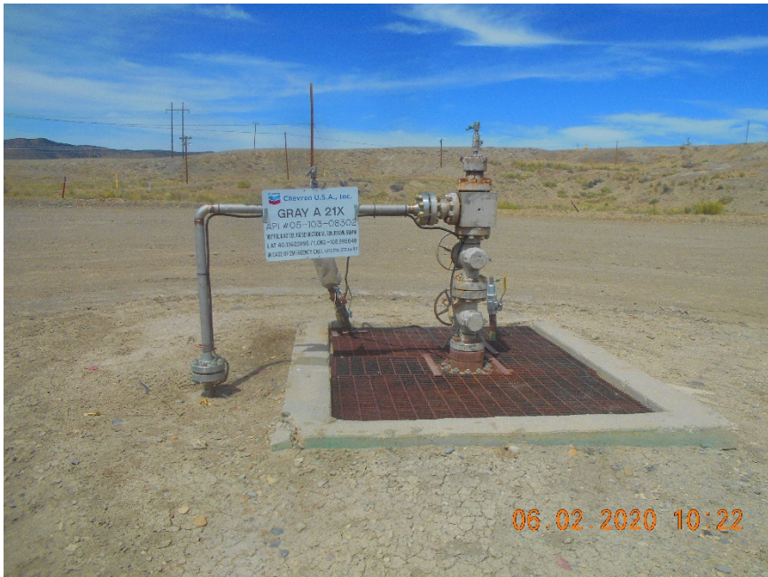
Injection wellhead
