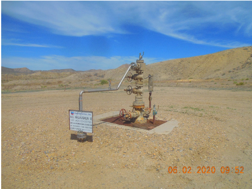
Injection wellhead
