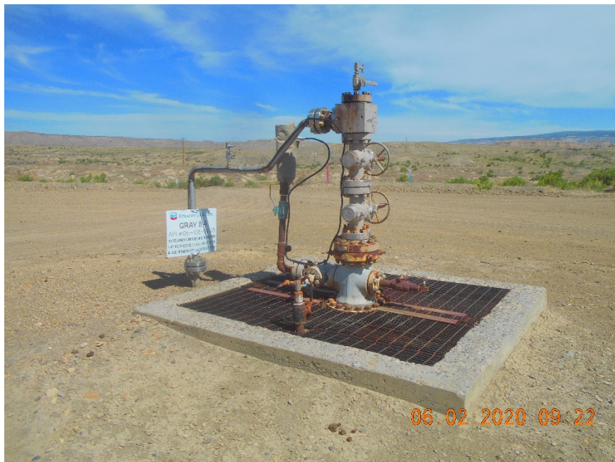
Injection wellhead
