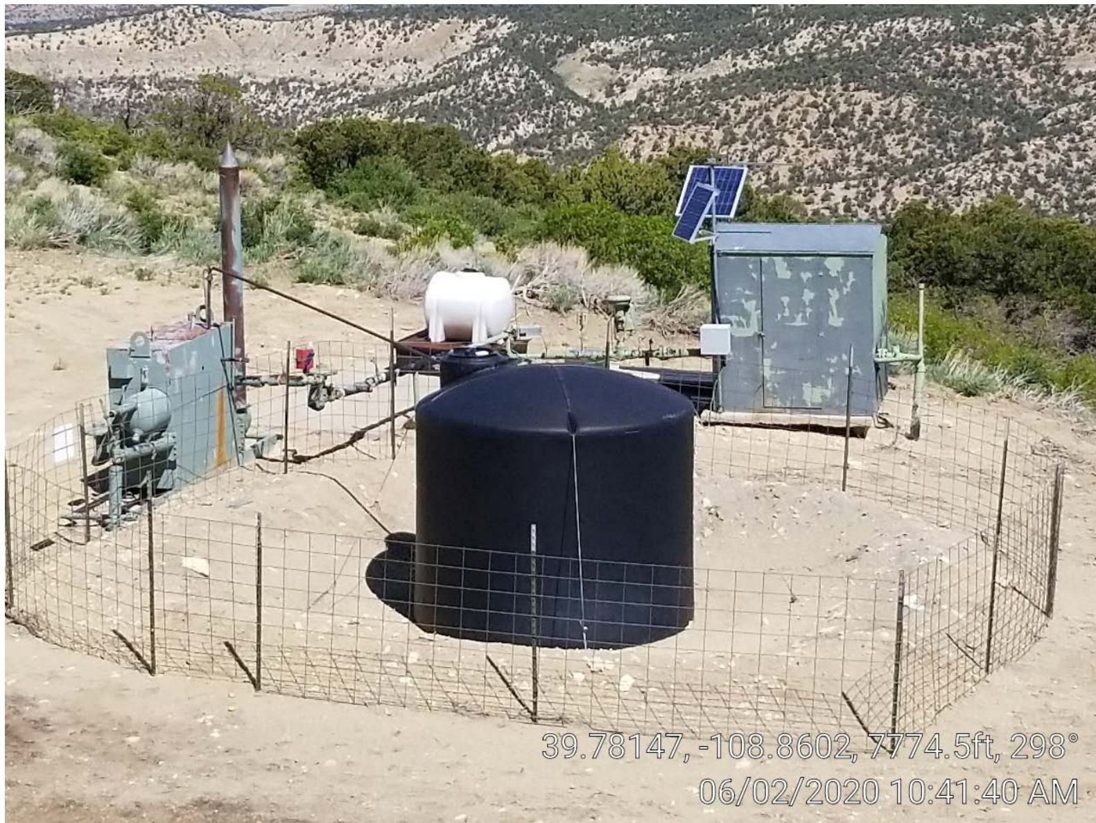
Photo 3. Separator, tank, and meter building.
