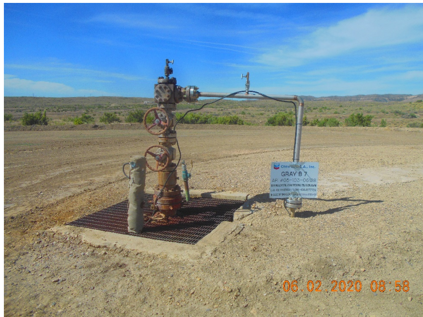
Injection wellhead
