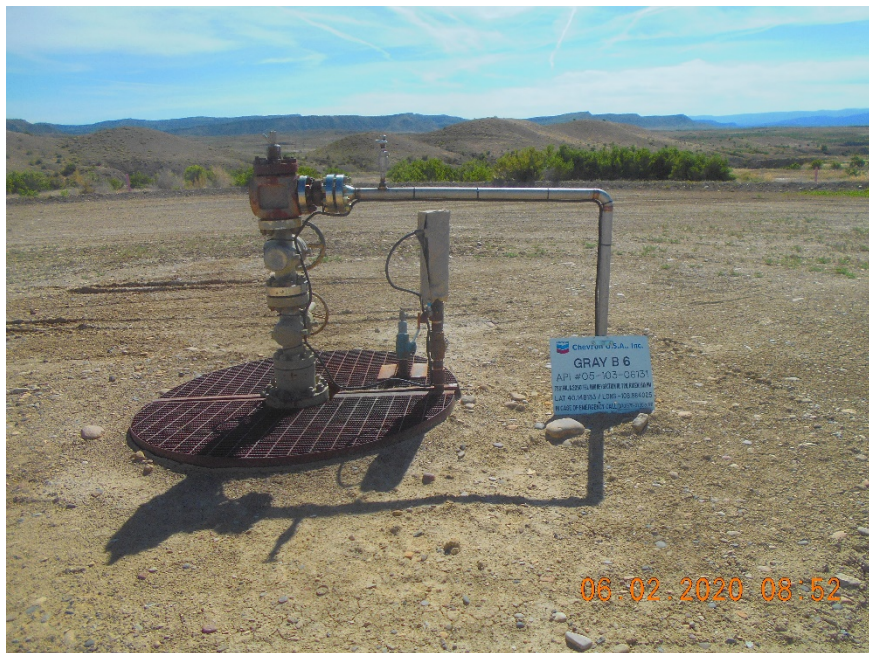
Injection wellhead
