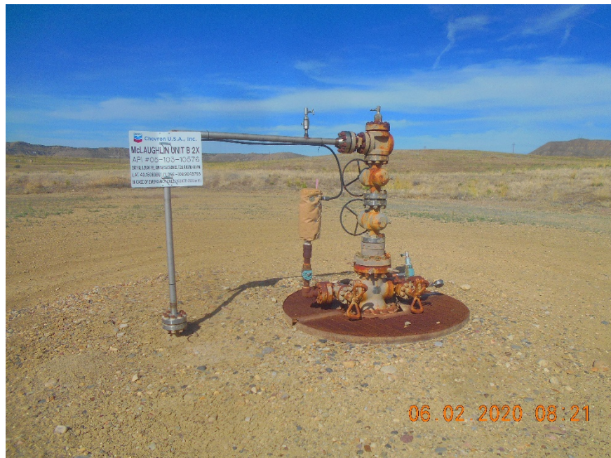
Injection wellhead
