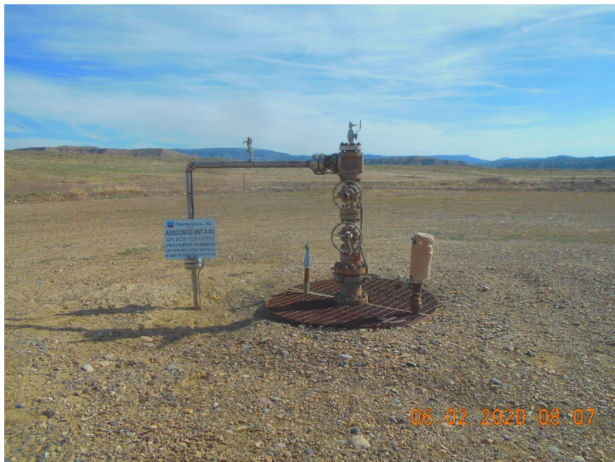
Injection wellhead
