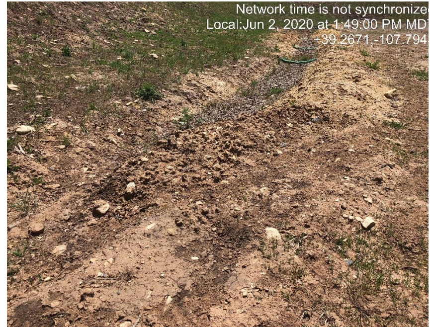
Photo #1298 Berm has eroded and migrated into adjacent ditch.
