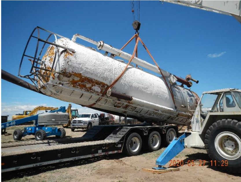
Photo 9: Loading treater on flatbed for haul off.
