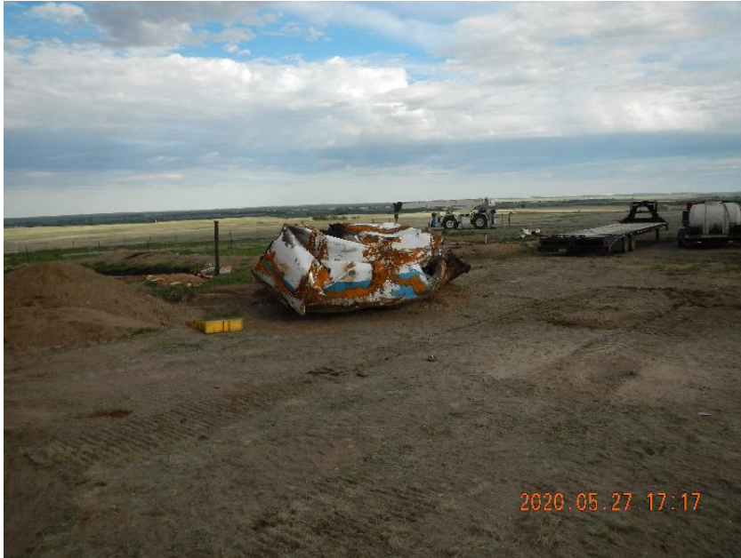
Photo 15: Crushed production tank ready for loading.
