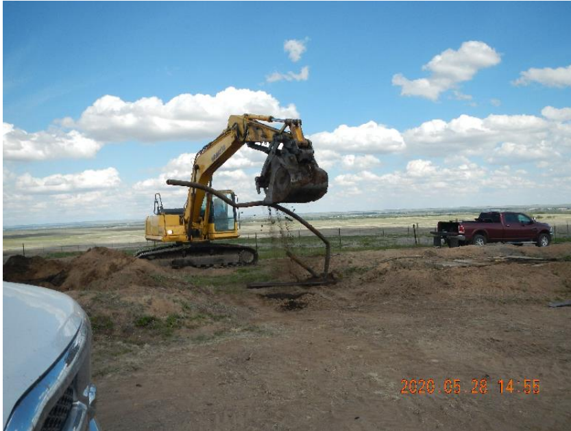
Photo 23: Excavating flow line.
