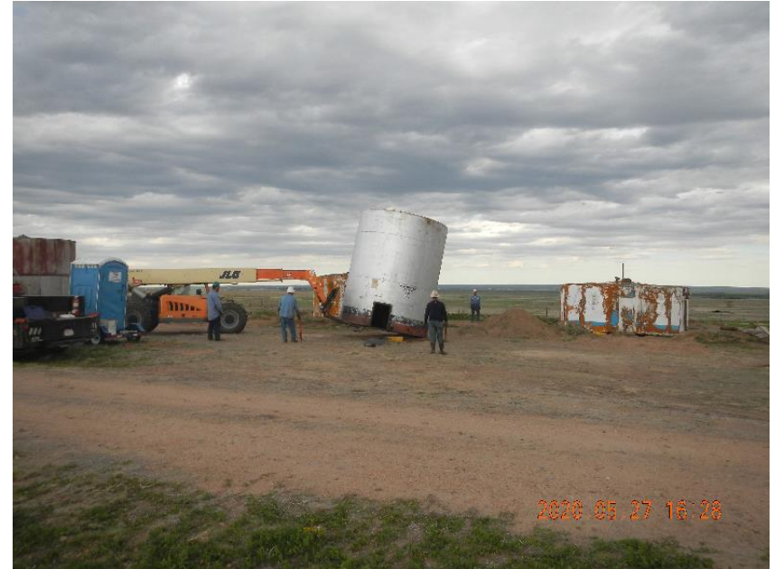
Photo 12: Laying down water tank for loading.
