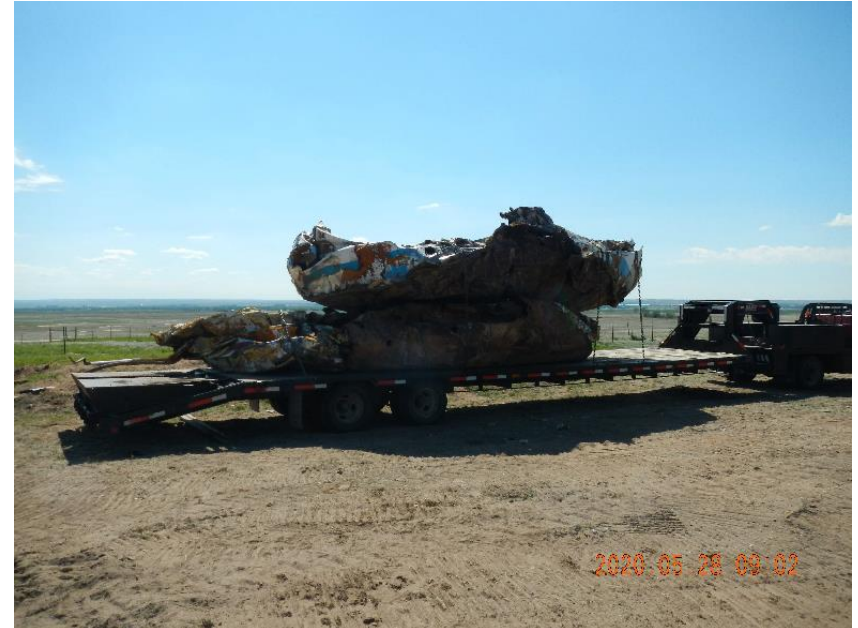
Photo 16: Loaded crushed production tanks leaving location.
