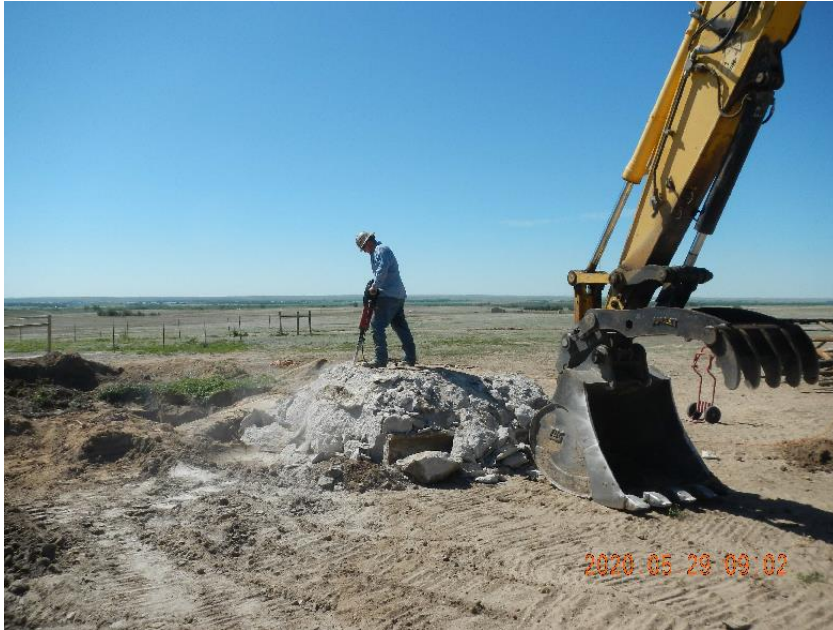
Photo 27: Jack hammering concrete treater base pad for removal.
