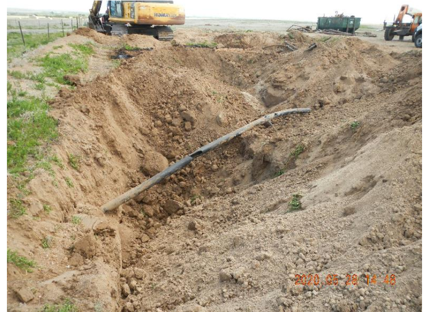
Photo 22: Removing flow line.
