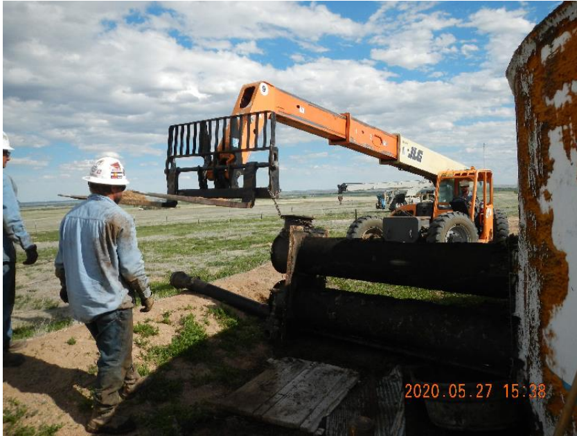
Photo 11: Removing flame tube from heated tank for haul off.
