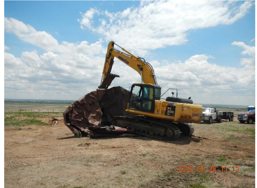
Photo 18: Rolling crushed production tank for loading.
