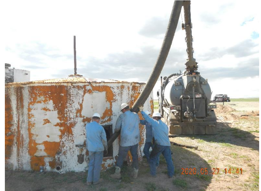
Photo 10: Crew using HydroVac to remove heavy fluids from production tank.
