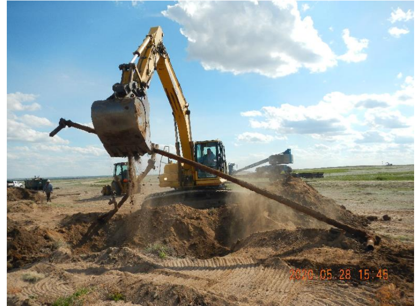
Photo 26: Excavating and removing flow lines.
