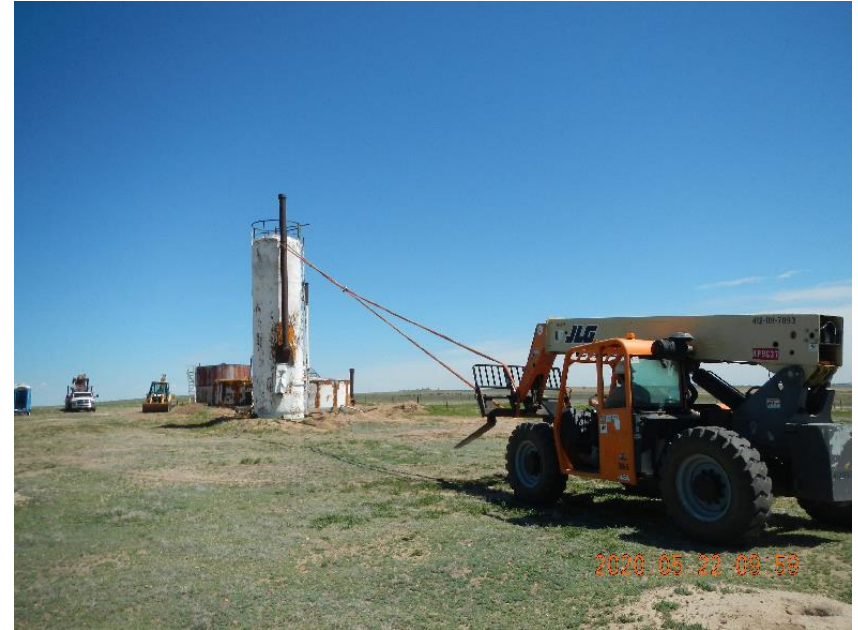
Photo 8: Laying treater down for removal.
