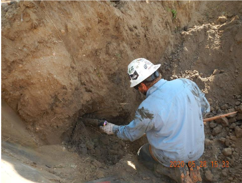
Photo 25: Cement plugging flow line.
