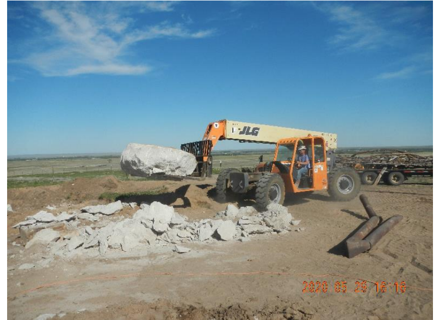
Photo 28: Loading concrete treater base pad for haul off.
