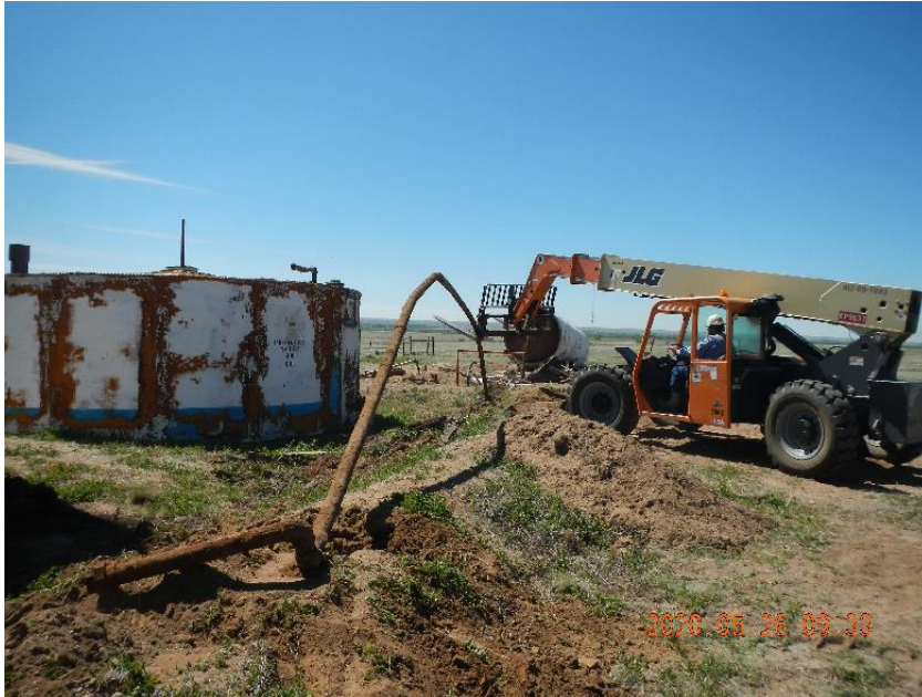
Photo 21: Removing flow lines.
