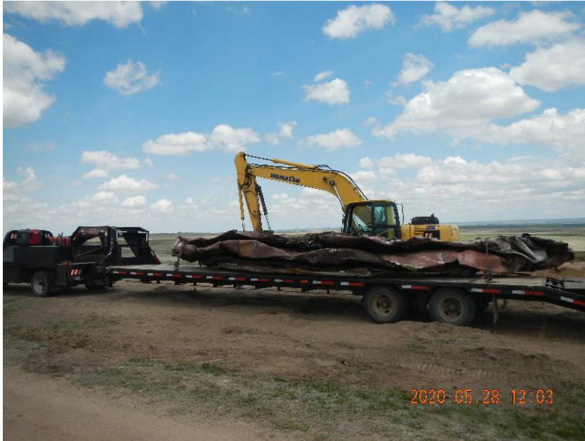
Photo 19: Loading crushed 1000 BBL tank for haul off.
