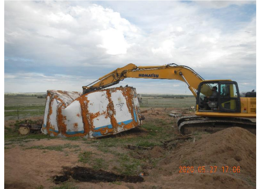
Photo 14: Crushing 300 BBL production tank for haul off.
