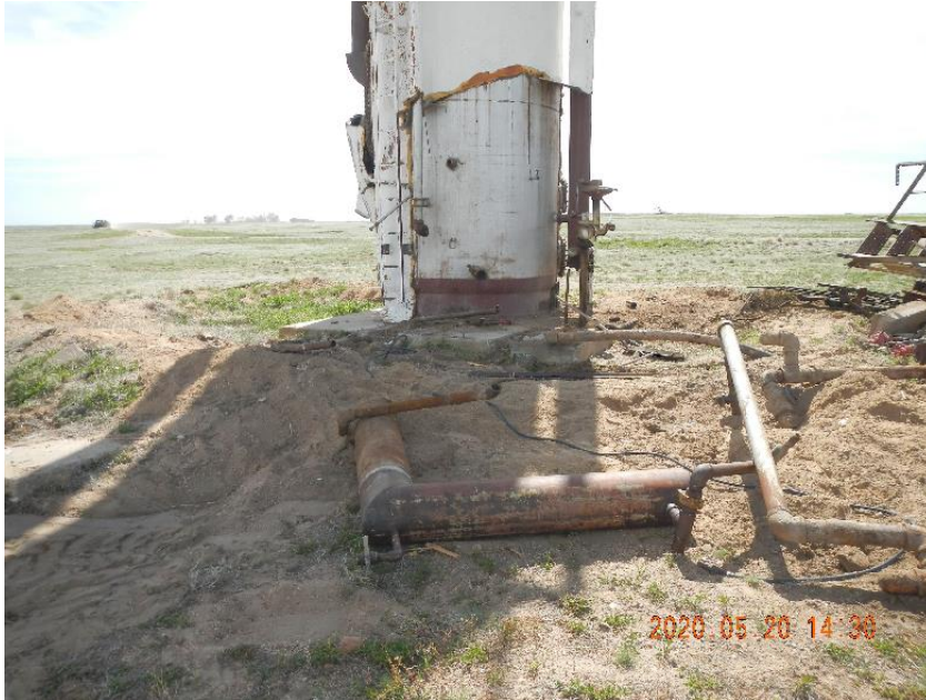
Photo 7: Treater shed torn down and removed flow lines.
