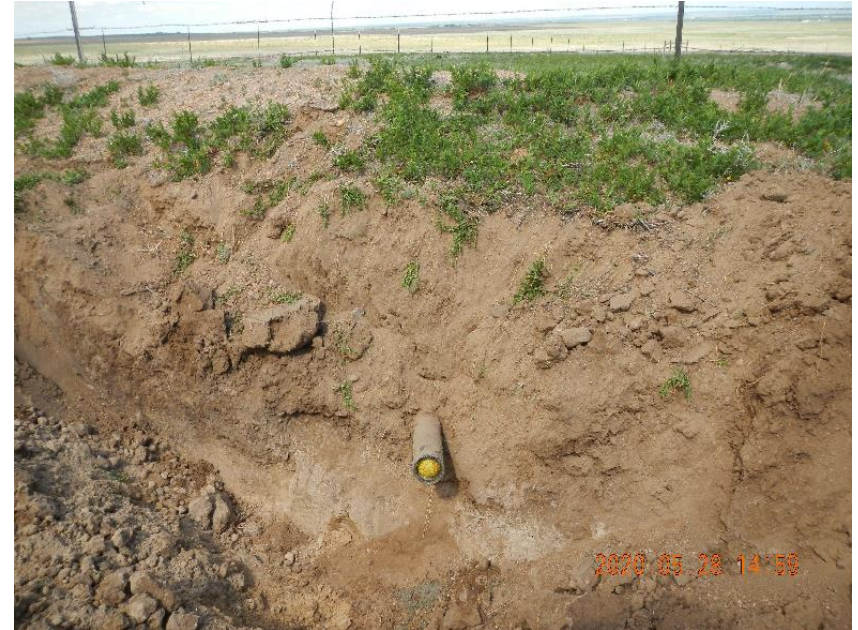
Photo 24: Cement plugged flow line. Foam ball in front of and behind cement to keep it in place.
