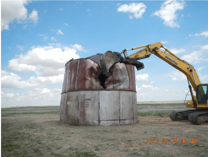
Photo 17: Crushing 1000 BBL production tank for removal.
