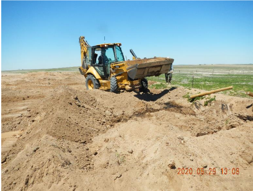
Photo 29: Berms for spill site being built.
