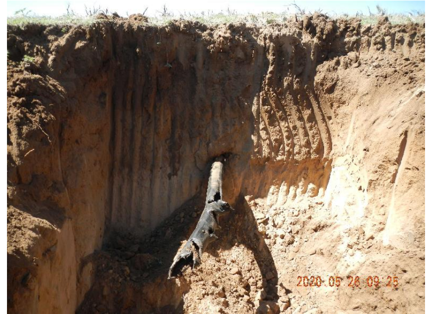
Photo 14: Excavated flow line.
