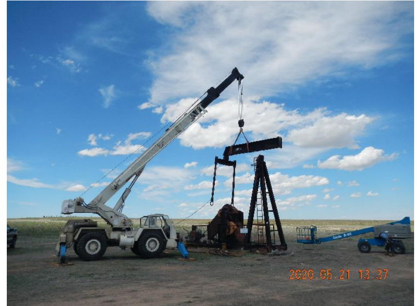
Photo 8: Removing walking beam and pitman arms from unit.
