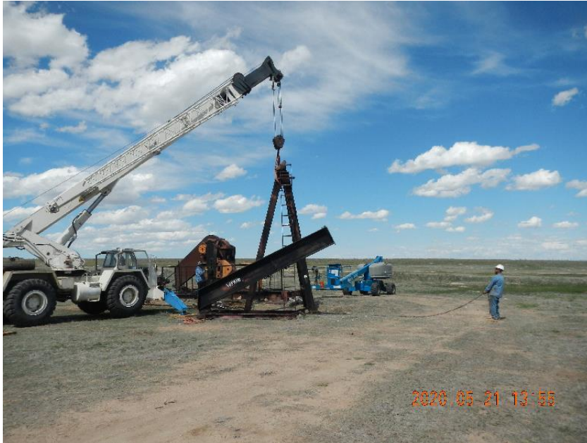
Photo 9: Sampson post removed from unit.
