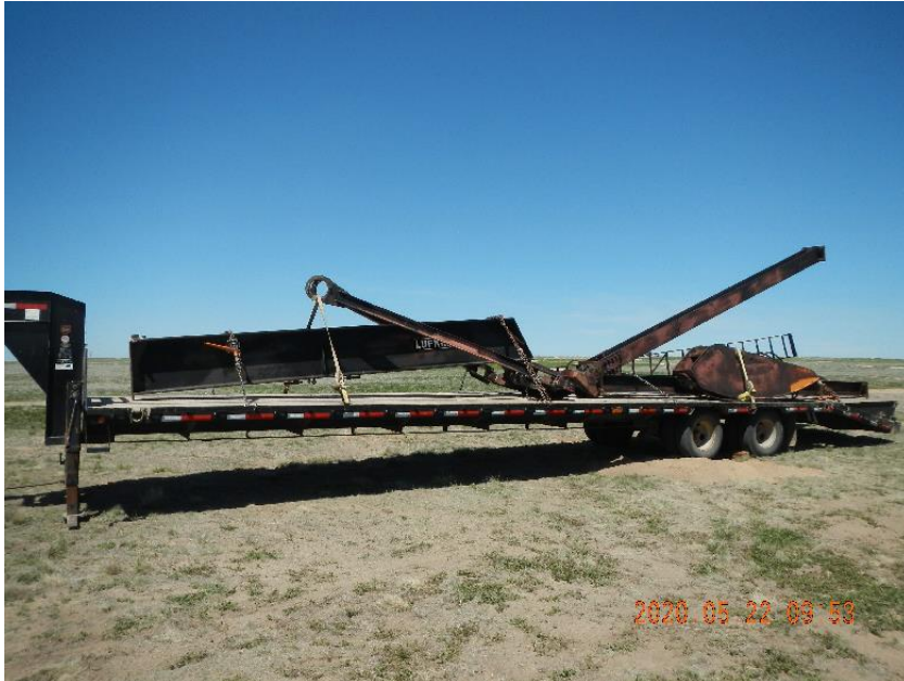
Photo 11: Walking beam, horsehead, and Sampson post loaded for removal.
