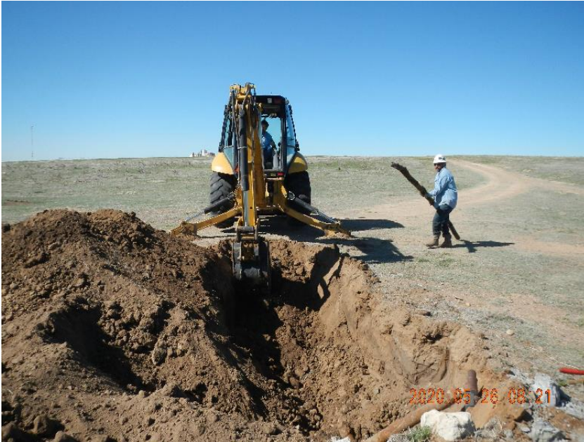
Photo 13: Excavating production flow line.
