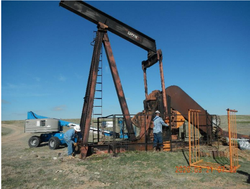
Photo 7: Crew breaking bolts loose to disassemble pumping unit.
