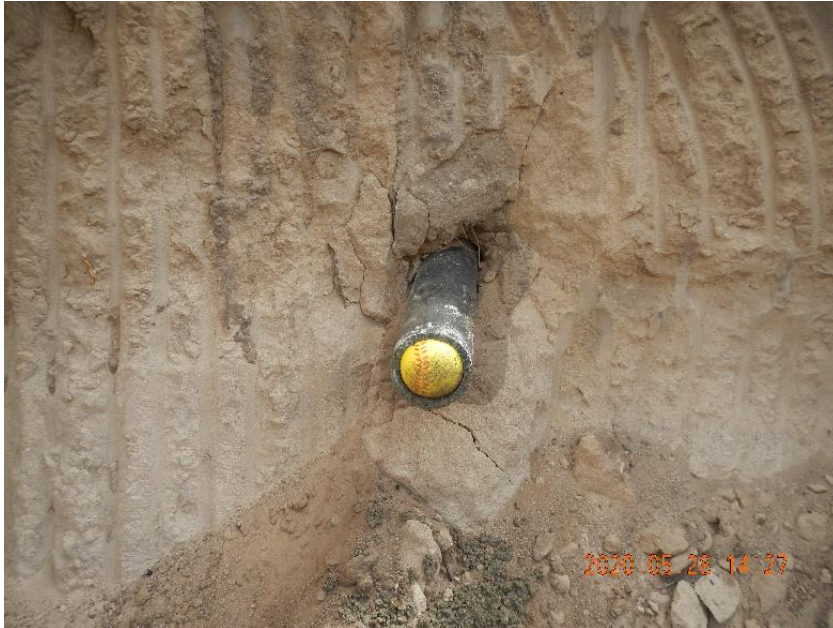
Photo 15: Flowline cut off and cement plugged. Foam ball placed in front of and behind cement to keep it in place.
