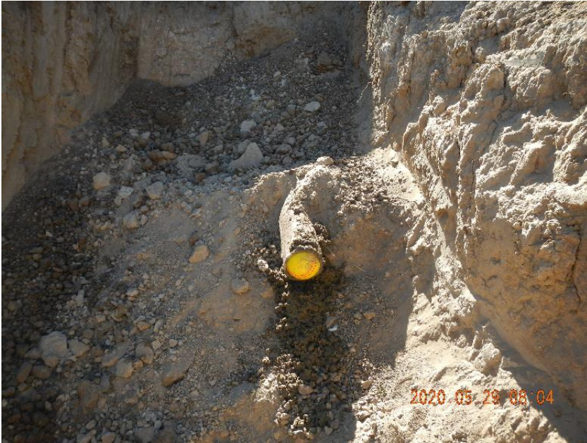
Photo 13: Cement plugged flow line. Foam ball inserted in front of and behind cement to keep it in place.
