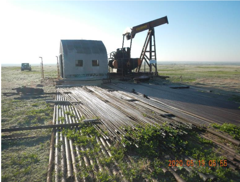
Photo 3: Rods and tubing left on site after well plugging.
