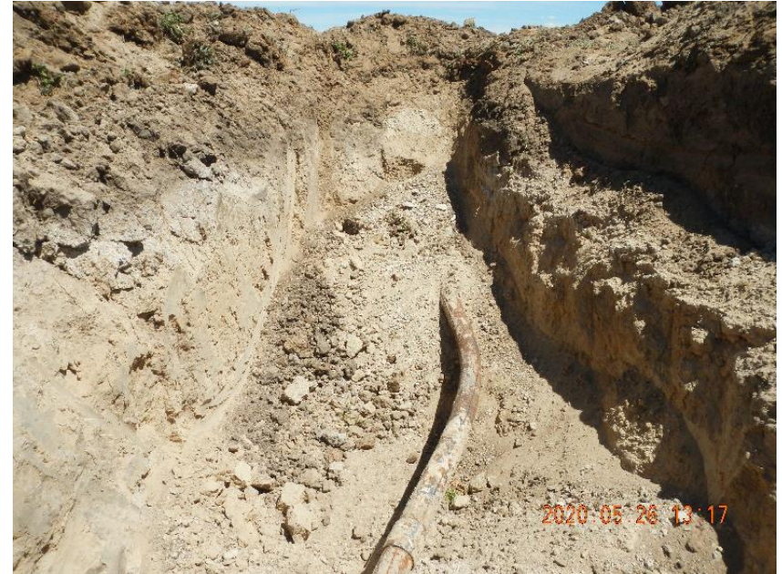
Photo 12: Excavated flow line.
