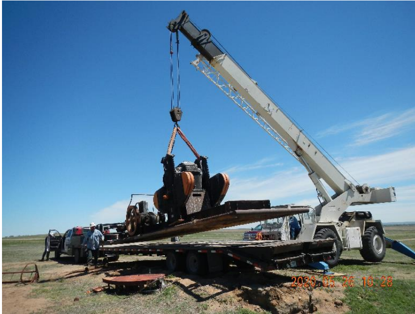
Photo 9: Loading pumping unit base for haul off.
