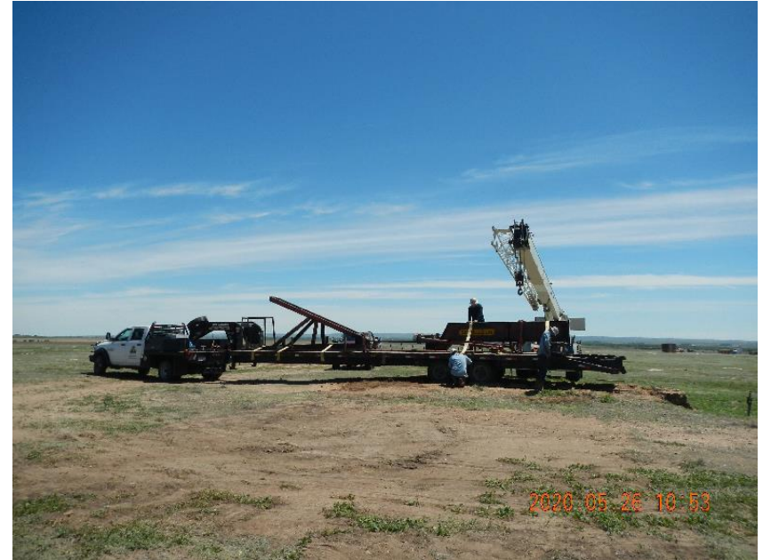
Photo 10: Loaded walking beam, horsehead, and Sampson post for haul off.
