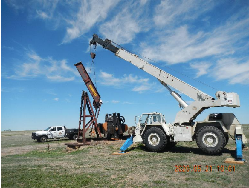
Photo 7: Removing walking beam and pitman arms from Sampson post.
