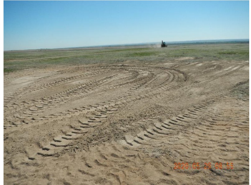
Photo 14: Backfilled and dressed site.
