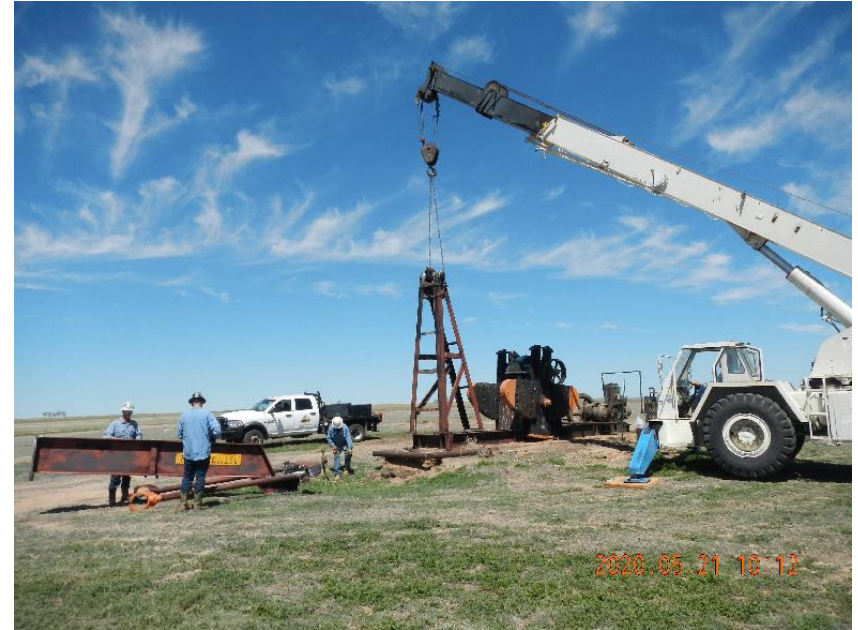
Photo 8: Removing Sampson post from pumping unit base.
