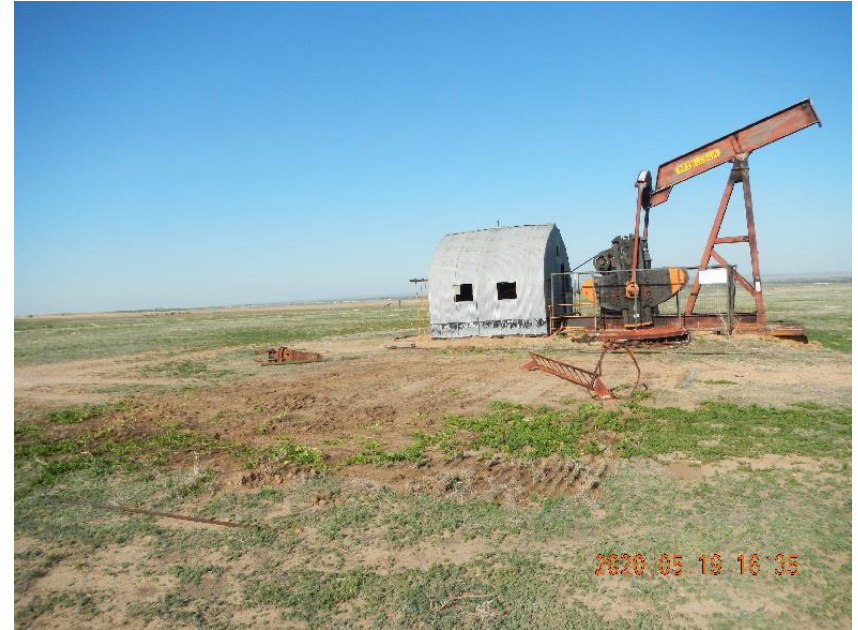
Photo 4: View of site after tubing and rods removed.
