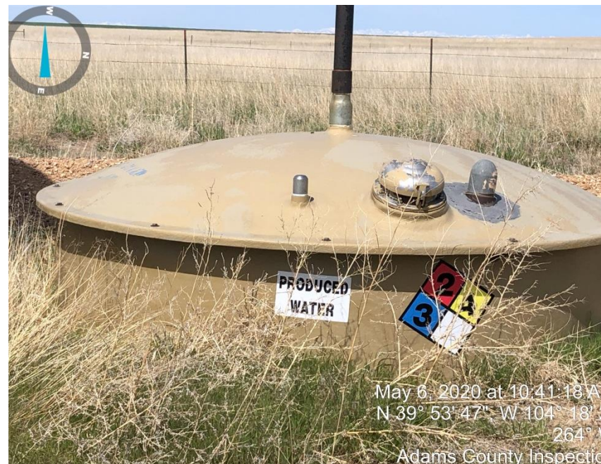
Photo#2 Corrective Action: No label showing amount tank holds.
