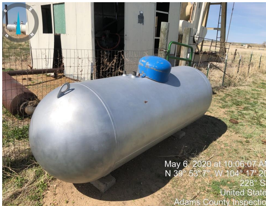
Photo#5 Corrective Action: Tank is unmarked
