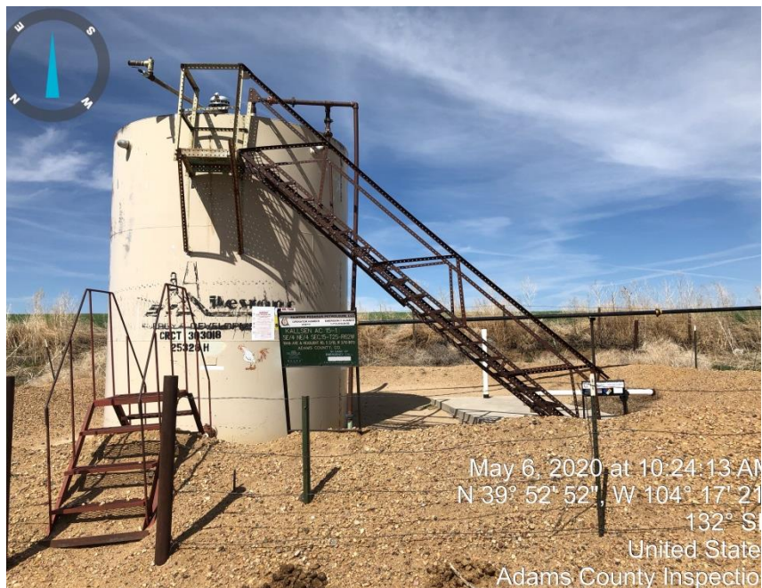
Photo#1 Production tank and produced water pit
