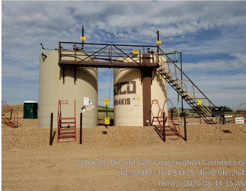
Photo #3 Tank Battery
