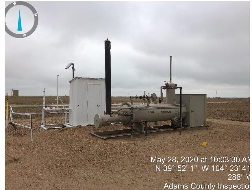
Photo #2 separator and meter run.
