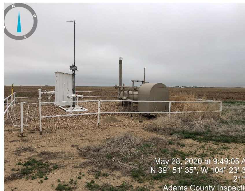
Photo #2 separator and meter run.
